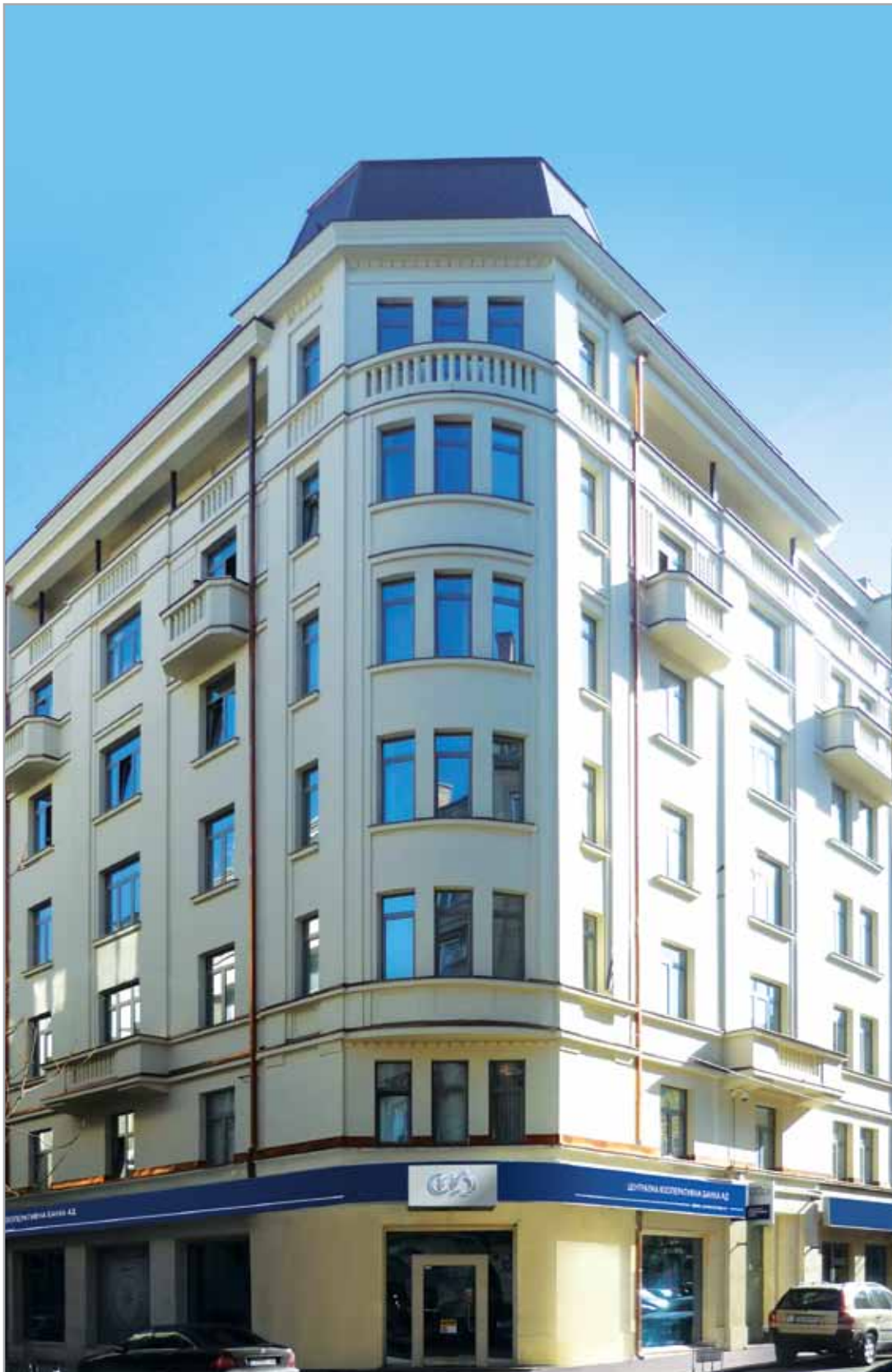
The main building of Chimimport, Sofia
