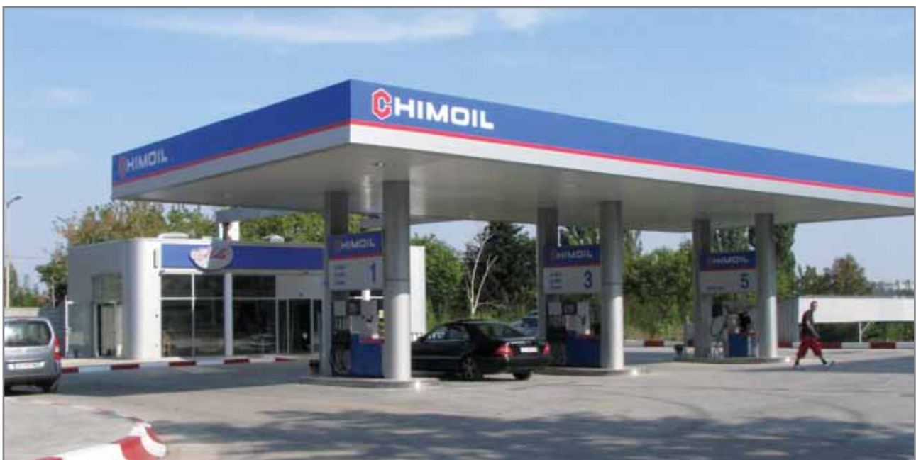
Chimoil BG Ltd filling stations
