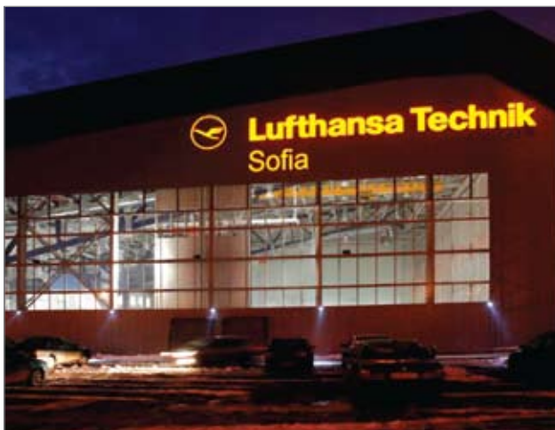
Hangar of Lufthansa Technik Sofia Ltd
