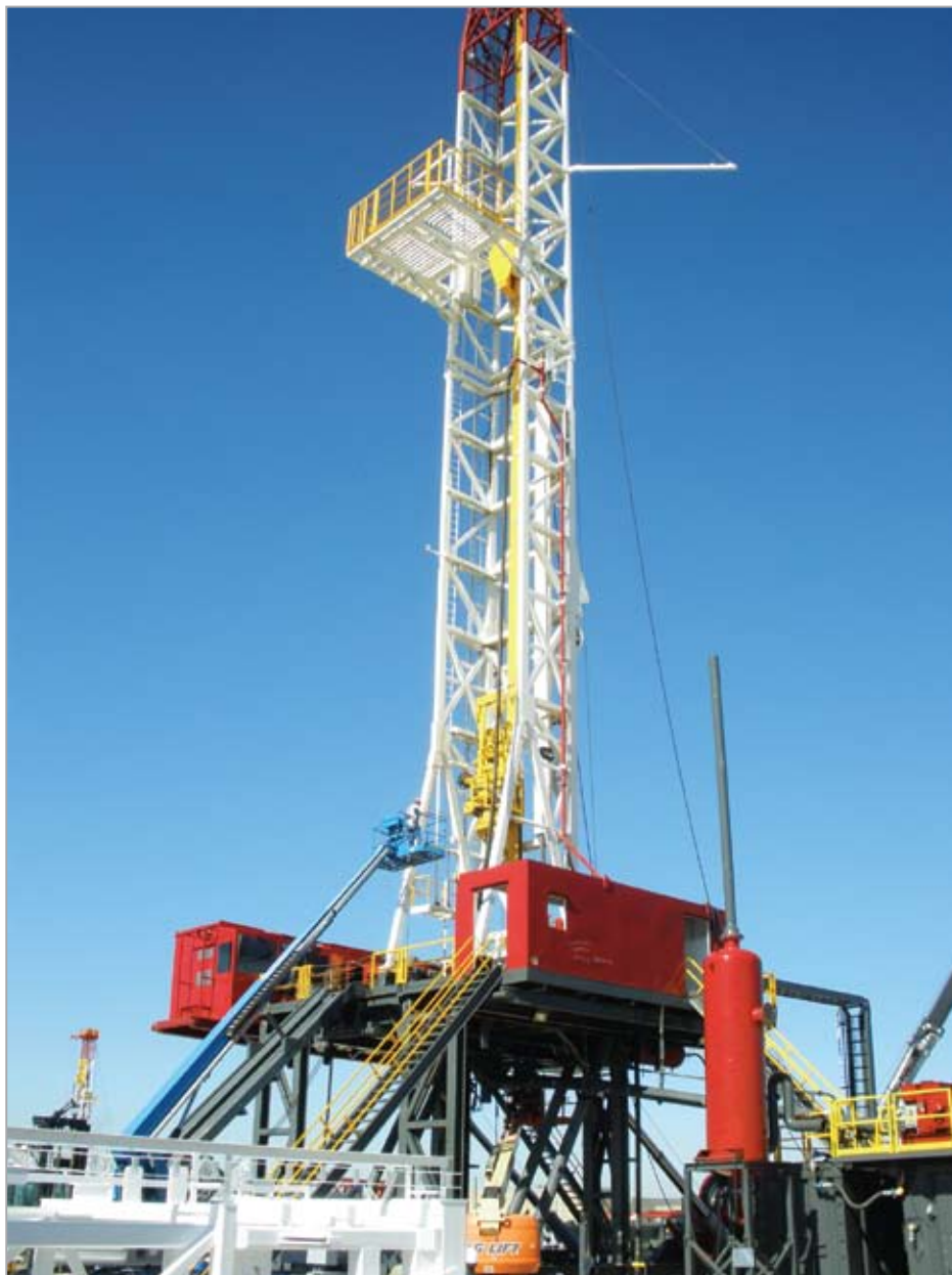
IDEAL - 1500 Drill Rig
