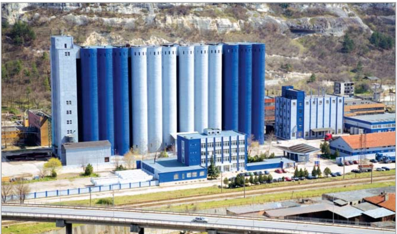
Food Oil Producing Plant, Provadia
