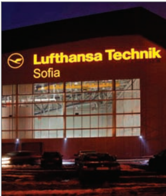
Hangar of Lufthansa Technik Sofia Ltd
